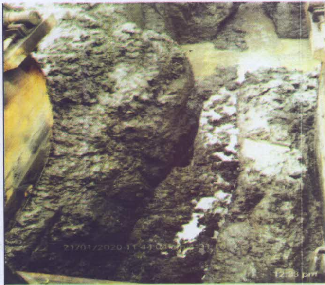
Figure 2: No impact on the pipeline.
