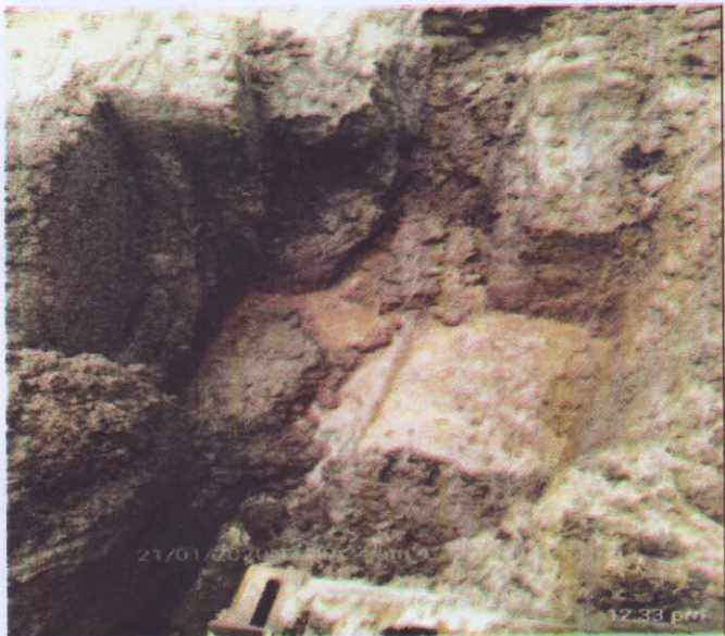
Figure 1: Excavation of the pipeline.
